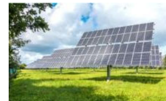
Solar Power Generation
