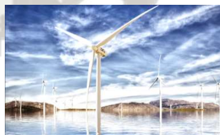
Wind Power Generation
