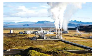
Geothermal Power Generation
