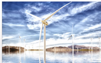
Wind Power Generation
