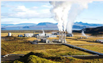
Geothermal Power Generation
