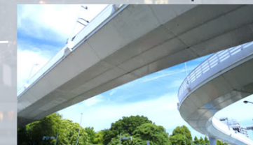
Large-scale Refurbishments of Three NEXCO Companies
