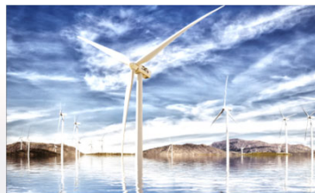
Wind Power Generation
