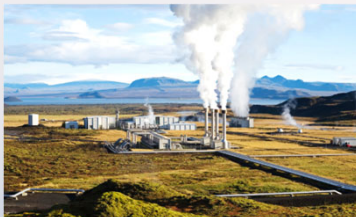
Geothermal Power Generation
