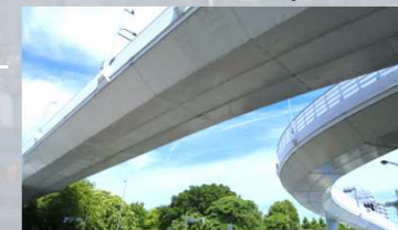
Large-scale Refurbishments of Three NEXCO Companies
