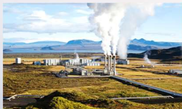
Geothermal Power Generation
