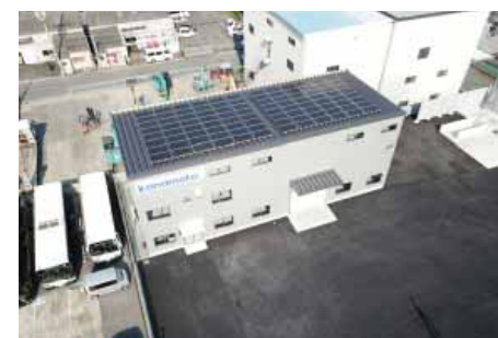
屋上に太陽光発電設備を設置した京都営業所 (2019年8月開設) The Kyoto Branch with solar power generation equipment installed on its roof (opened in August 2019)
